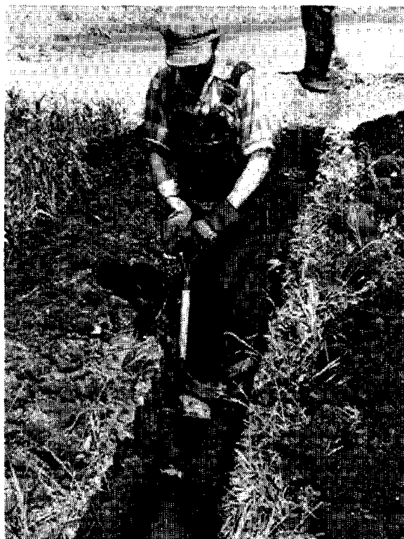
Trenching with a spade
