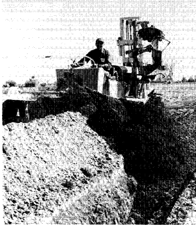
Backfilling with machinery
