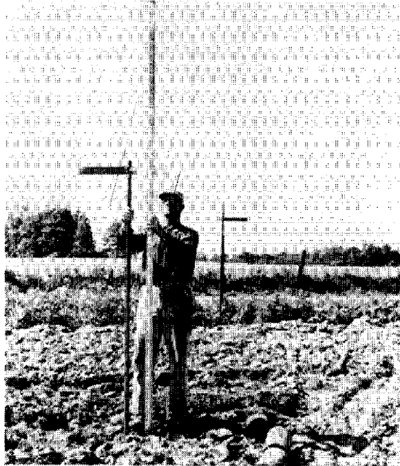
Setting targets for a trenching machine
